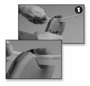
Step 1. Use plastic tubing cutters to cut the tubing between the pointed ends of the repeating 1" SharkBite imprint pattern. The pattern provides a visual aid to determine if the tube has been inserted all the way into the fitting. Ensure the tube is cut square. A square cut end allows the tubing to be inserted all the way into the fitting. Ensure the tube has no rough edges, cuts or abrasions (rough edges, cuts or abrasions may damage the O-ring and cause the fitting to leak).
