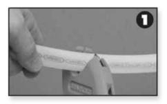
**Step 1.** Use plastic tubing cutters to cut the tubing to length, making sure that you have a good square cut. A rough or uneven cut will result in a weakened joint.
