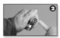
Step 2. SharkBite fittings come with integral tube support liners. Ensure that the support liner is in place. The liner reinforces the wall of the PEX tubing to help prevent collapse of the tubing wall.
